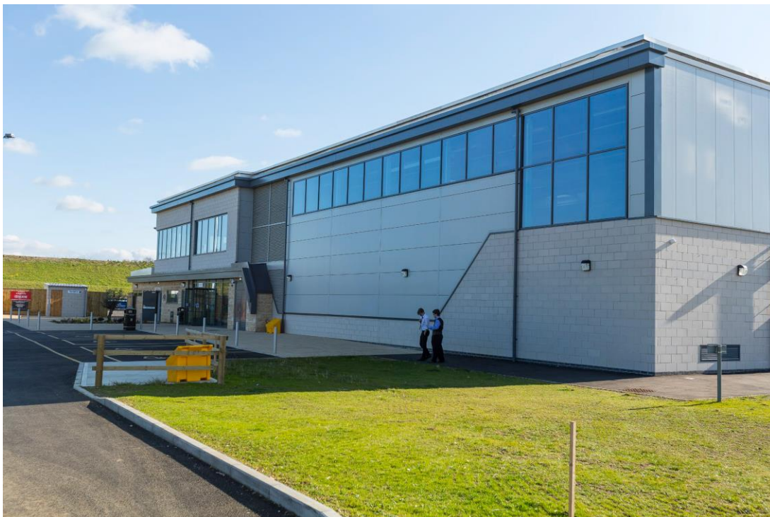
Existing building face to which the new extension will added
